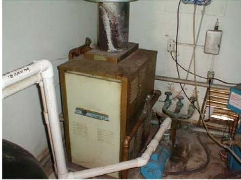
The pool contractor advises the 400K Teledyne Laars pool heater is original and is in poor condition.
